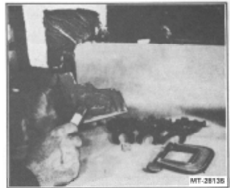
Figure 37. - Applying Epoxy Adhesive
