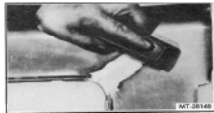
Figure 54. - Filling Repaired Surface
